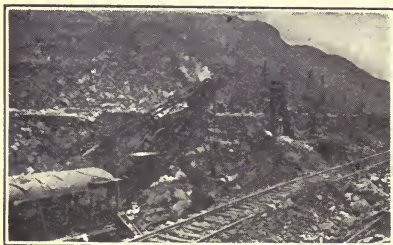
STEAM SHOVELS AT WORK ON THE PANAMA CANAL CULEBRA CUT MAY 20, 1913
